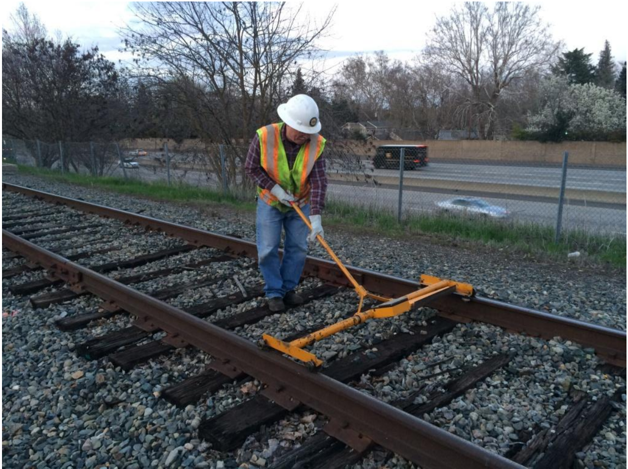
Mike H. uses the gauge-measurer to measure the track's gauge near MP 2.6
